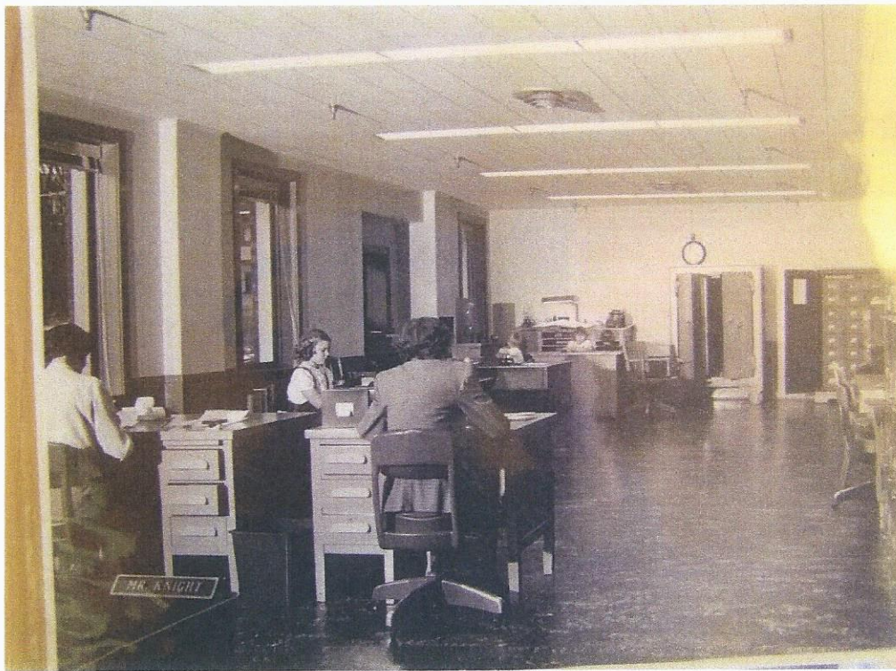
Figure 15: c. 1950 photograph of the renovated interior of 86 St. Paul Street
